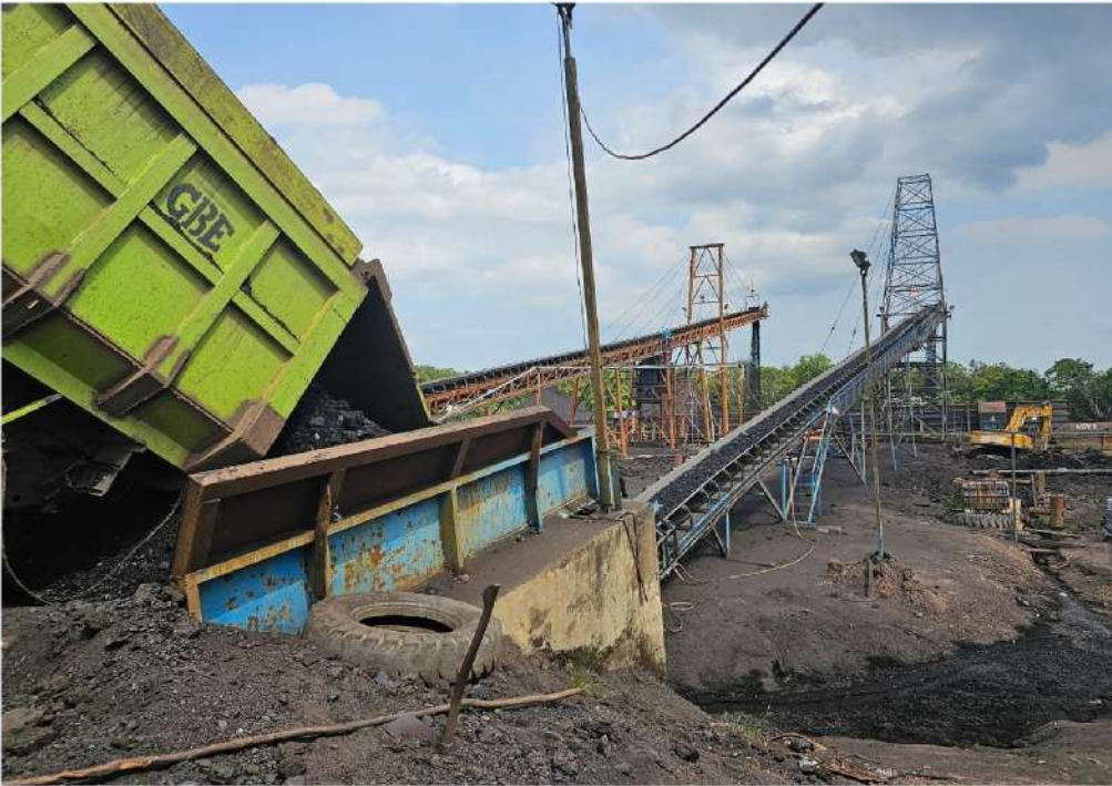
Loaded Truck along with coal dropping to conveyor belt.
