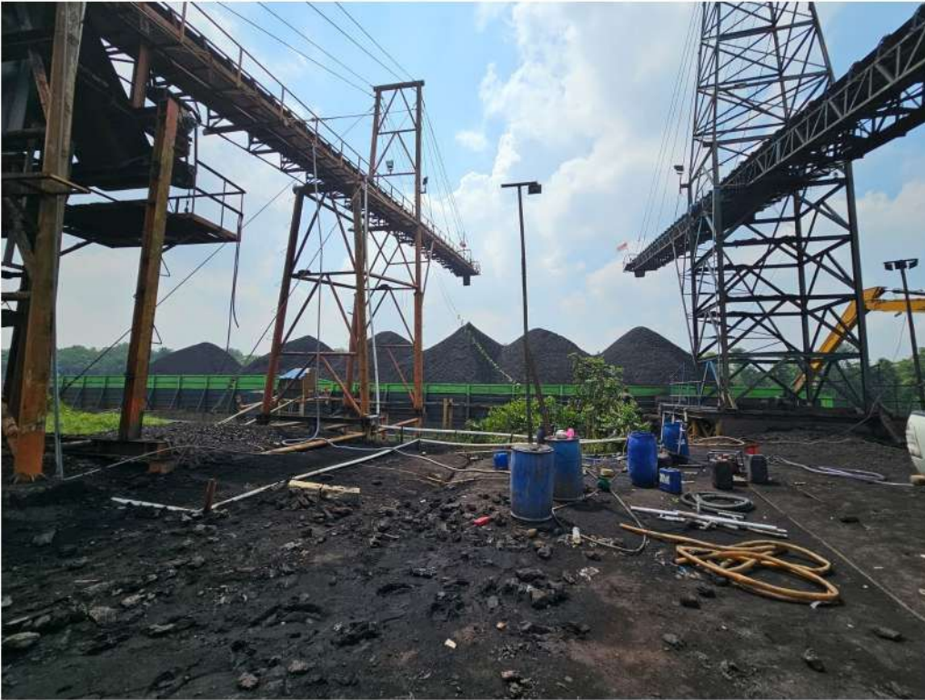
Coal loading from Jetty to Barge through conveyor belt
